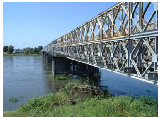
Temporary Nile Bridge
