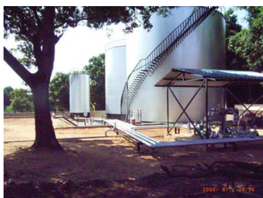
New Fuel Tanks
