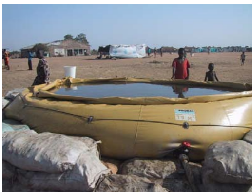
Temporary Tank for Water Selling
