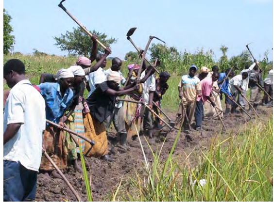
Canal construction by farmers
