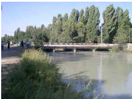
No.15(1)橋梁全景
