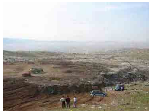
Rehabilitation of Compacted Landfill Area by Soil Covering
