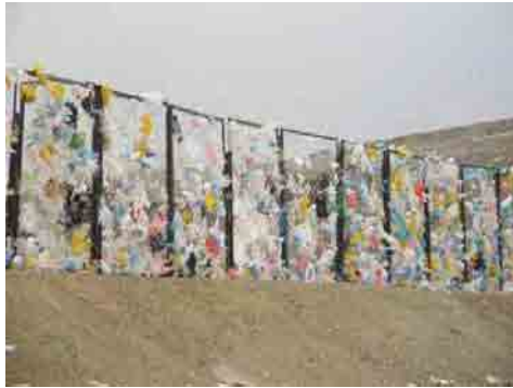
Prevention of Waste Scattering by Movable Fence
