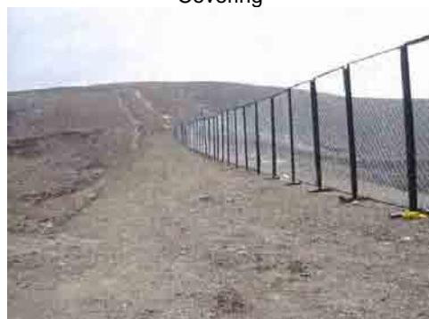
Movable Fence for Prevention of Waste Scattering
