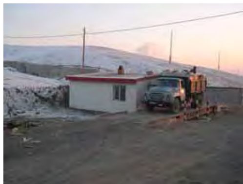
<Weighbridge> The weighbridge, which was installed at the gate, measures the weight of waste every time a collection vehicle enters the disposal site.
