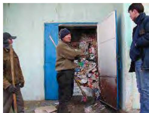
High-rise apartments have a dust chute. Waste collected through the dust chute is stored in a storage room. Waste is stored long and often causes odor and breeding of vermin.
