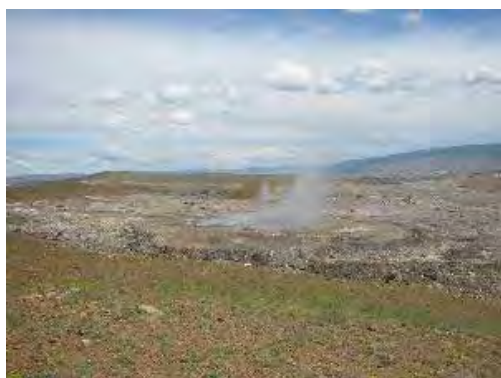
<Ulaan Chuluut Disposal Site, June 2005 > The UCDS is the largest one in UB, and 90% of the generated waste in UB is disposed of here.
