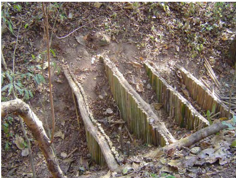
Small dams made with local material (bamboo)
