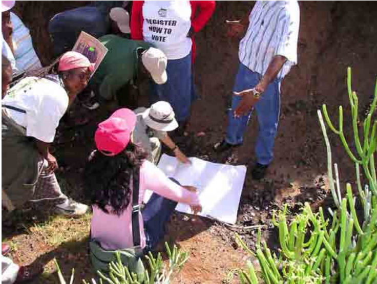
Construction of a check-dam at a village in South Africa, South African Policy Research Project (April 2006)
