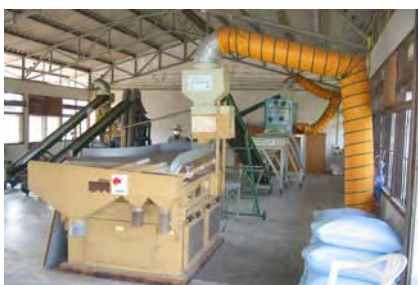
Equipment supplied from the Project at KKANRDC (Gravity separator)
