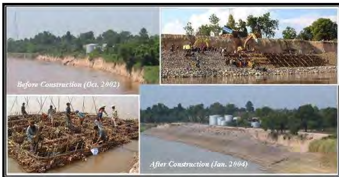
Figure 9.4.2 Construction of Pilot Works at Ban Dongphosi Site
