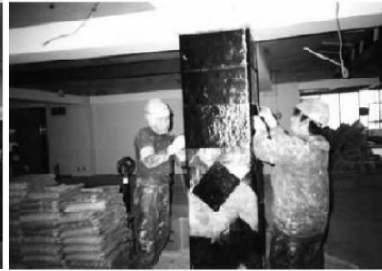
Carbon sheet jacking
