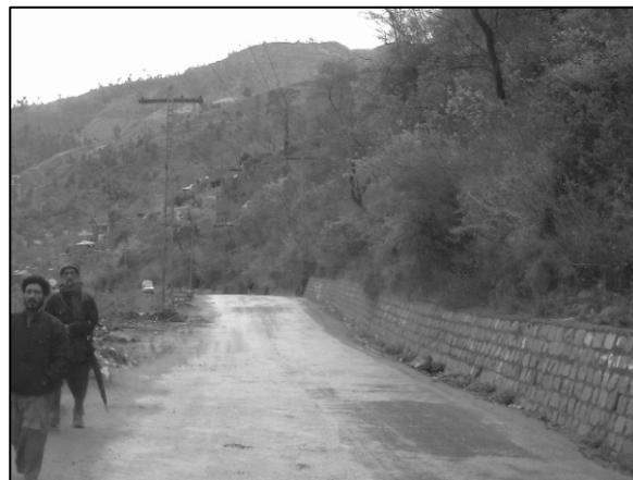
Photo-2a Landslide Hazardous Place in Chela Bandi Bridge - Alama Iqbal Bridge Road
