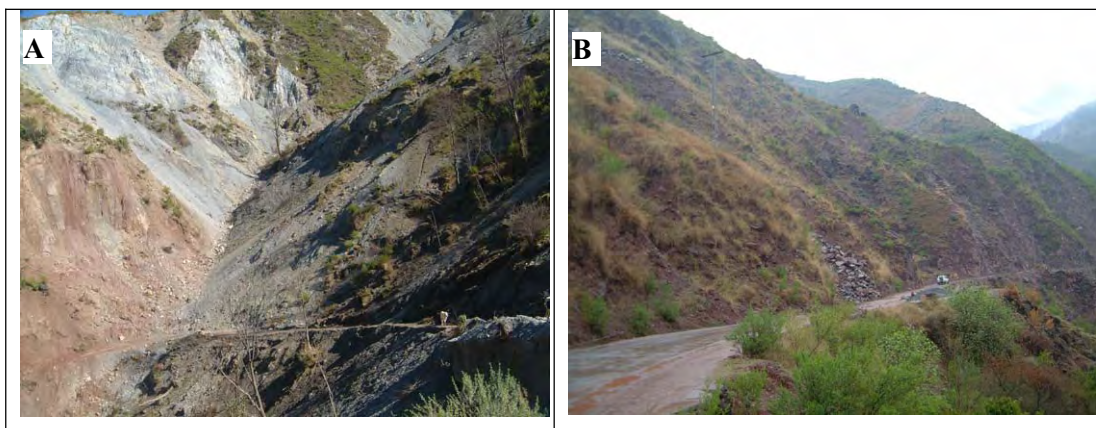
Figure 3.1.7 Rock Mass Collapses Occurred on Limestone (A) and Sandstone and Shale (B).
