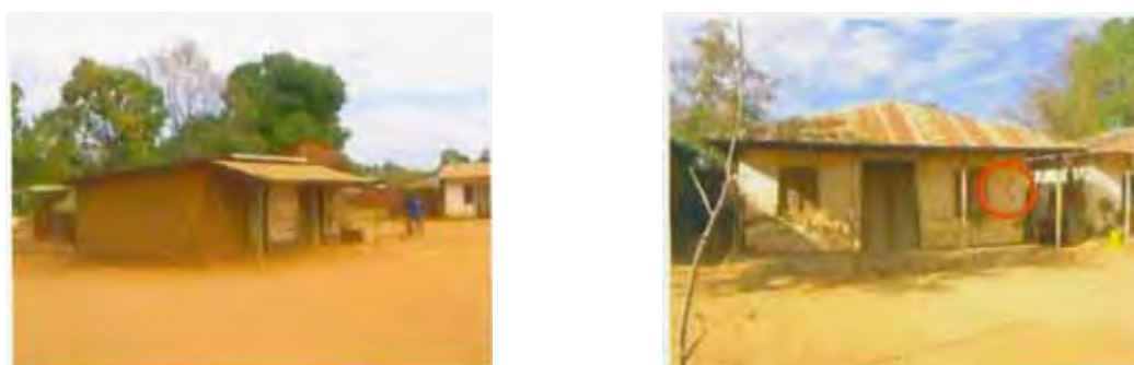
Photo 1.3 Houses inside the Existing Right of Way (ROW)
