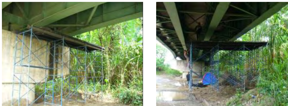
Figure 10.2.22. Scaffolding for Working Stage
