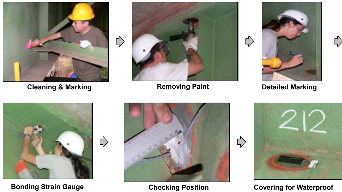
Figure 10.2.24. Strain Gauge Setting
