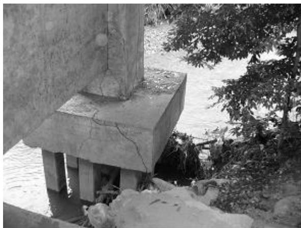
Figure 10.3.1. Scoring of Riverbed on No.16 Nuevo Bridge
