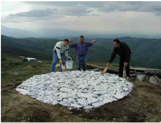
Installing Photo Signal (Photo Control Point Survey)
