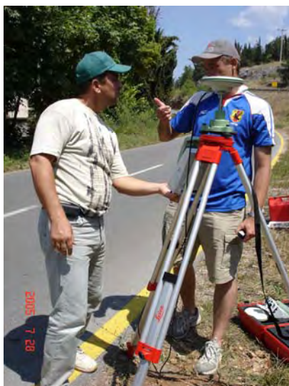
Technology Transfer (GPS Survey)
