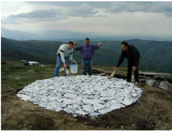
Installing Photo Signal (Photo Control Point Survey)
