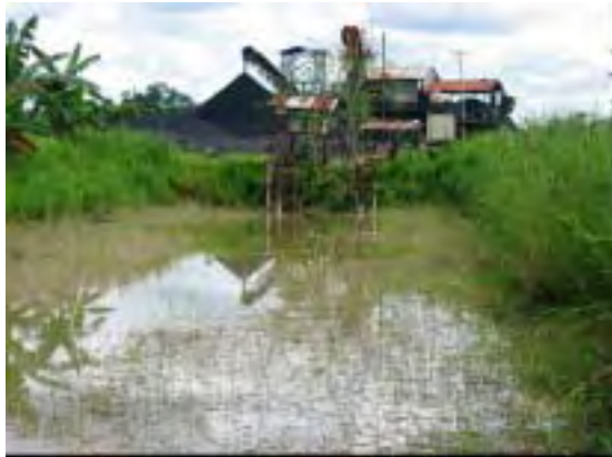
Photo 5-2-3 Facility Designed to Recycling Water
