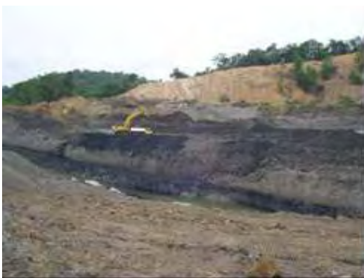
Open Cut Mine for Ash Disposal
