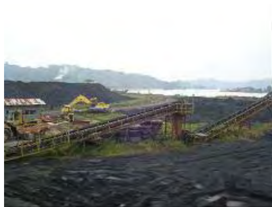
Old Coal Export Facilities
