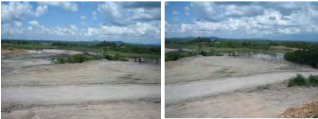
Photo 4-2-5 Reclamation of Settling Pond
