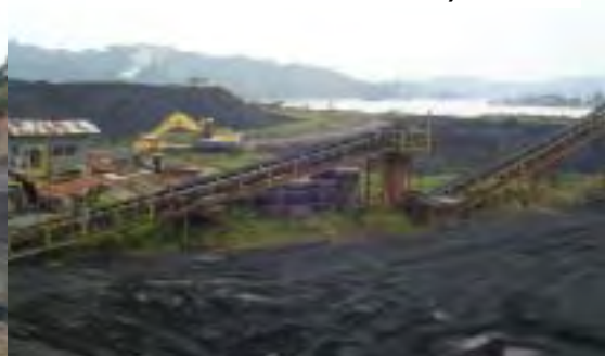
Old Coal Export Facility Area (Proposed Power Plant Construction Site)
