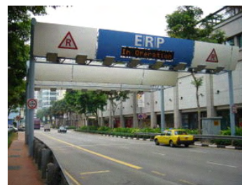
Figure 11.4-15 Electronic Road Pricing System
