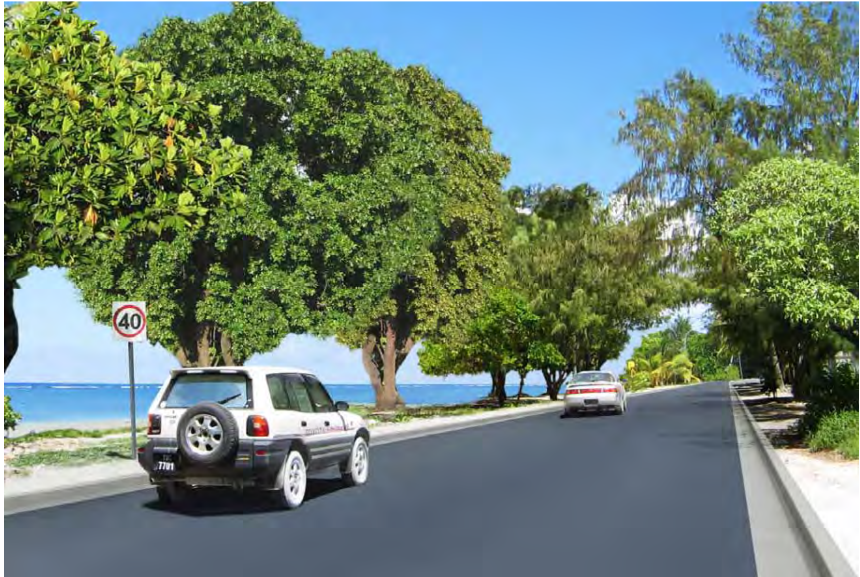
View of the Completed Road
