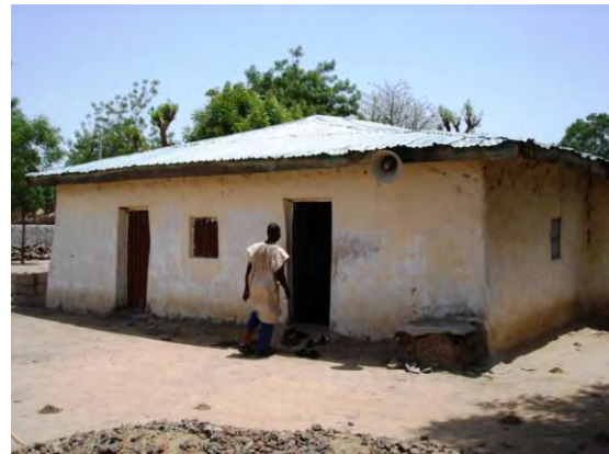
4) PF (mosque): Twelve (12) units of 15 W fluorescent lights are installed inside. They use an audible speaker as a DC load (10 W).
