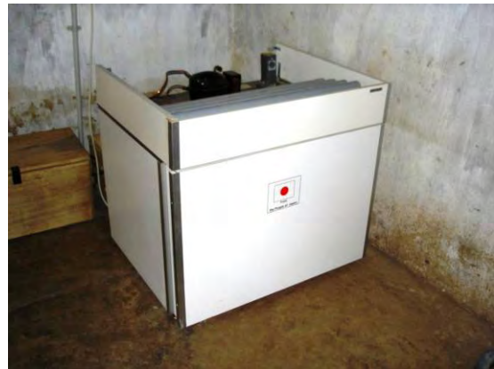
4) PV vaccine refrigerator: The refrigerator is certified by WHO and has a storage capacity of 38.7 liter. The inside of it is divided into freezer and cold storage.
