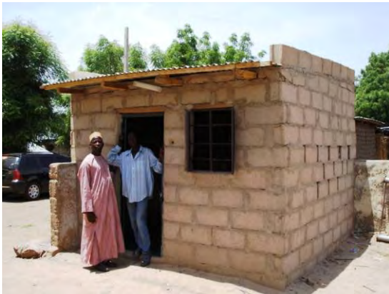
1) BCS Station (external): The villagers constructed the house by themselves.
