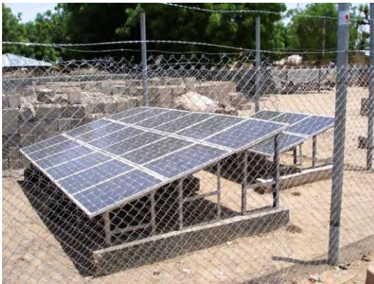
3) PV array: The array for BCS has a nominal maximum output 1,080 W comprised of eighteen (18) units of 60 W module (front). Meanwhile, the output of the array for PF is 360 W comprised of six (6) units of 60 W (back). The arrays face due south and their tilt angles are 15°.
