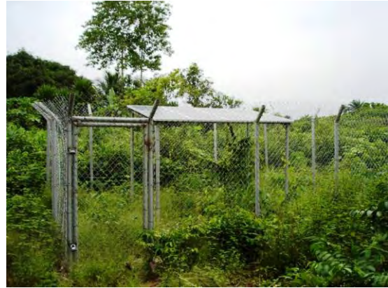
2) PV array: The array has a nominal maximum output 496 W comprised of eight (8) units of 62 W. The array faces due south and its tilt angle is 15°.
