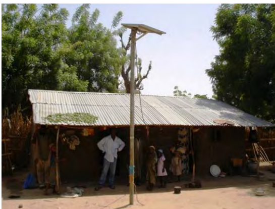
5) SHS: The PV module is as the same as for BCS (60 W). Two (2) units of 15 W fluorescent lights and a DC outlet are installed inside. The storage battery is sealed type with a capacity of 65 Ah.
