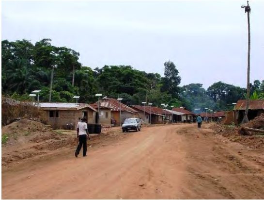
1) Center of Oke-Agunla Village: The houses are located along the street from north to south. The poles for SHS and SL are installed beside the houses.
