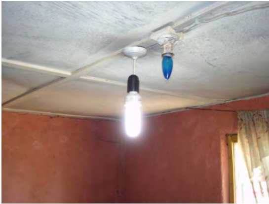
3) Lighting for SHS: The lighting (CFL) has expected lifetime of 5,000 hours and more.
