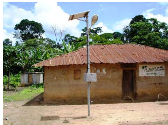
6) SL: The specifications of the equipment are as the same as in Jigawa. Considering the solar irradiation, the light turns on and off automatically and can be used for 4 hours a day (3 hours from sunset and 1 hours before sunrise).
