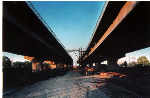
Delhi- Gurgaon Road Under Construction
