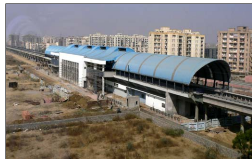
Metro Station under construction (Dwarka-10)
