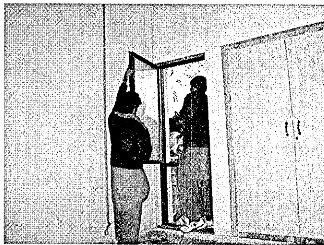
AL WIMDOW INSTALLATION
