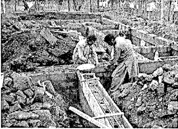
Nov 18 2006 Plinth Beam work
