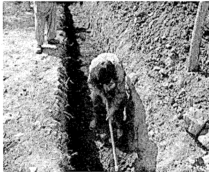
⑤ Nov 8 2006 Excavation Work
