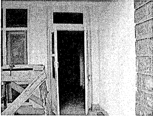
DEC14 2006 MO HOUSE RENOVATION: Painting Work
