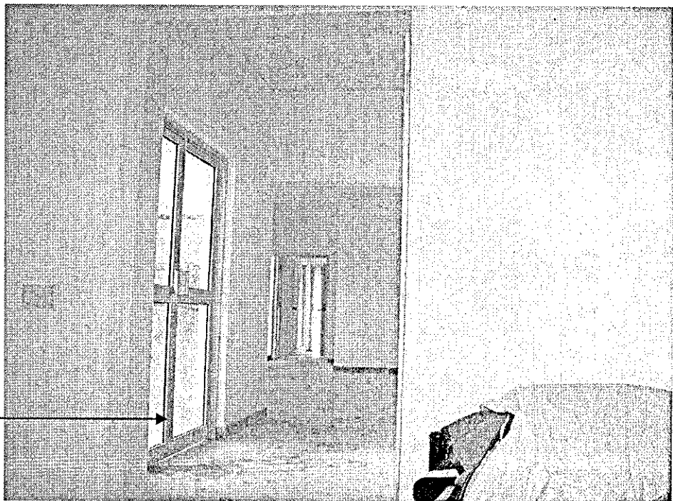
Upper Building Interior finishing
