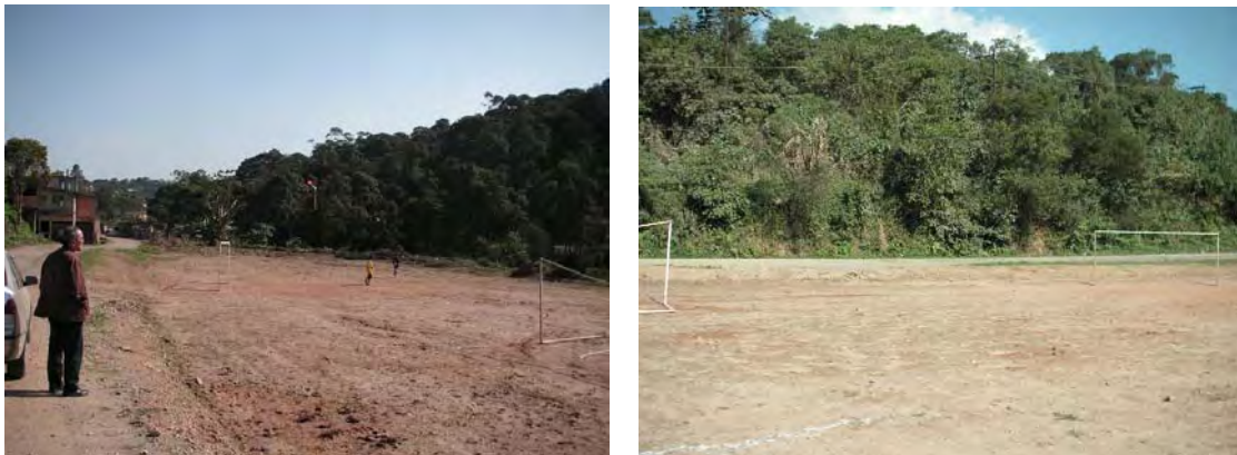
Photo 31.2.1 Project Site of Sewage Treatment Project in Santa Cruz
