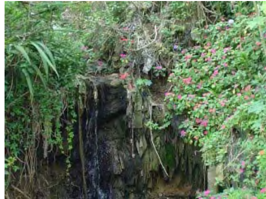
Photo 15.2.7 Exit of Leachate Discharge
