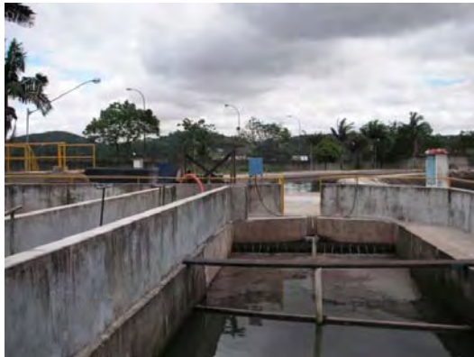
Photo 15.2.2 Riacho Grande WWTP
