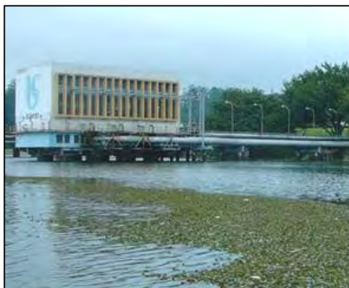
Photo 5.1.3 Aquatic Plant around Intake P/S
