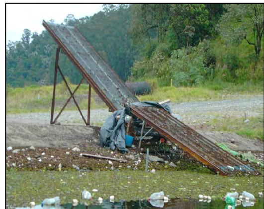
Photo 5.1.4 Belt Conveyor for Removal of Aquatic Plant
