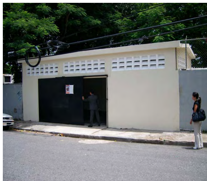
Temporal storage for common waste
