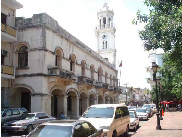
Consistorial Palace (Municipal Palace) in Colonial City
