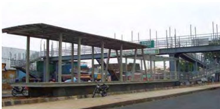
Figure A25.16 Station Under Construction in Jakarta
