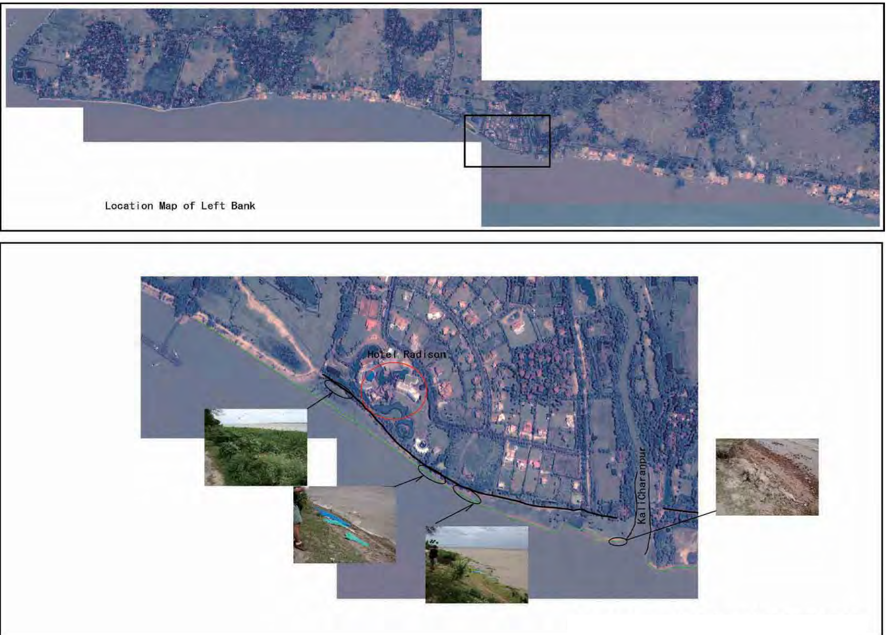
Figure 6.2.6 River Bank Protection Works at Left Bank (4/6)
