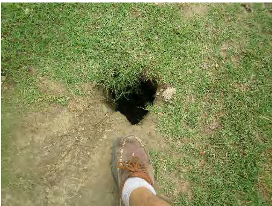
Figure 5.2.2b Initial stage of erosion possibly caused by the existence of dispersive clay.
