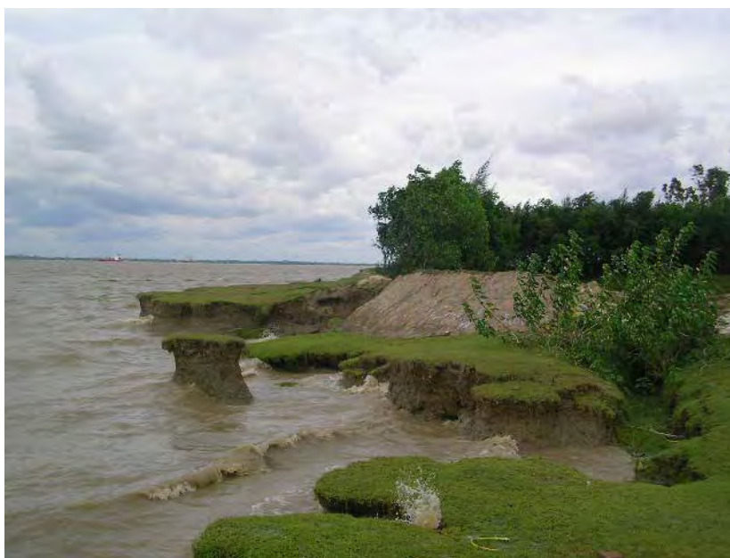
Figure 5.2.5a On-going Riverbank Erosion in the Hugli River
