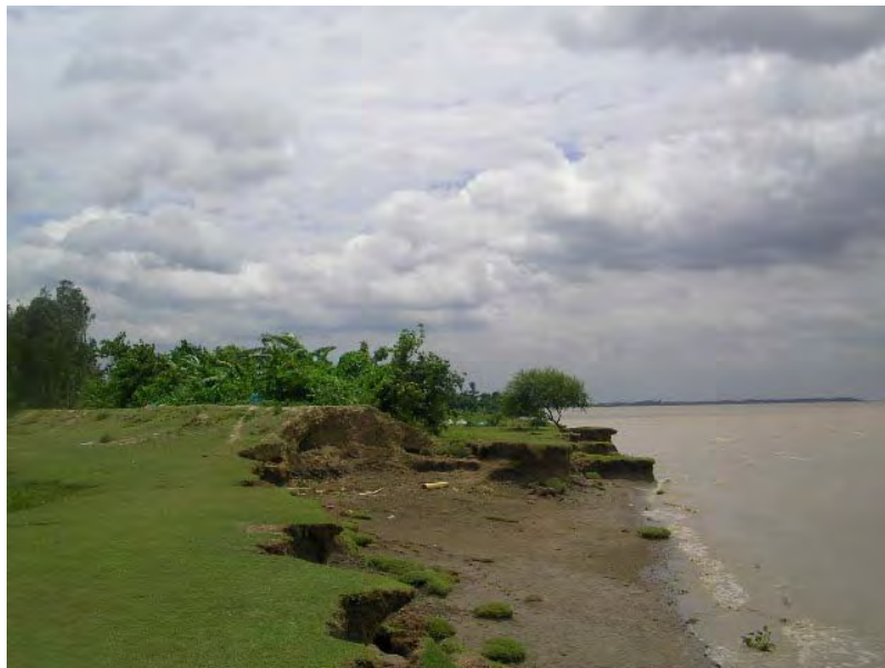
Figure5.2. 9 Damaged River Bank
