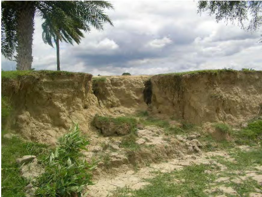
Figure 5.2.2a Erosion of a riverbank due to the possible existence of dispersive clay
