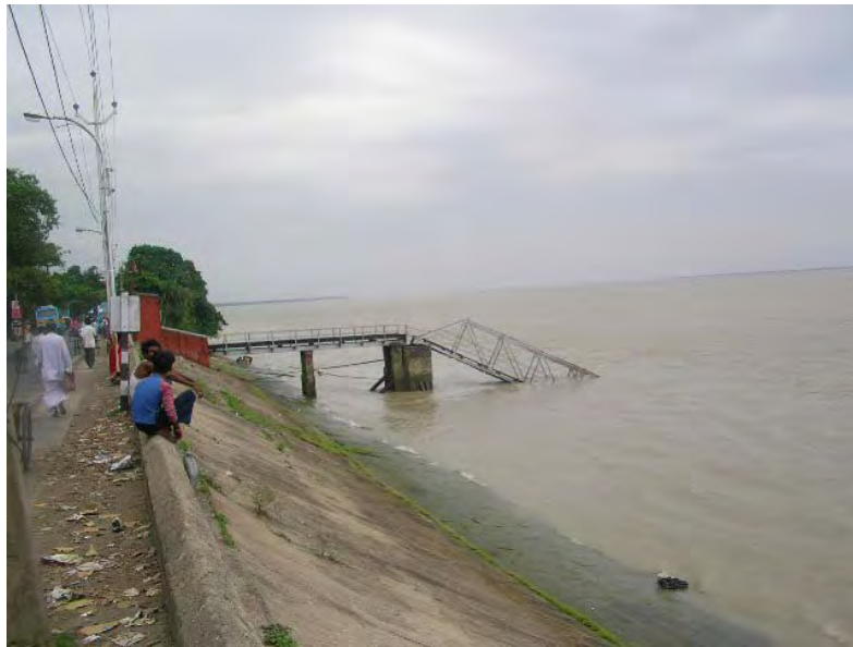
Figure 5.2.8 Damaged Ferry Pier in Diamond Harbour (photo taken on 8 July 2006)
