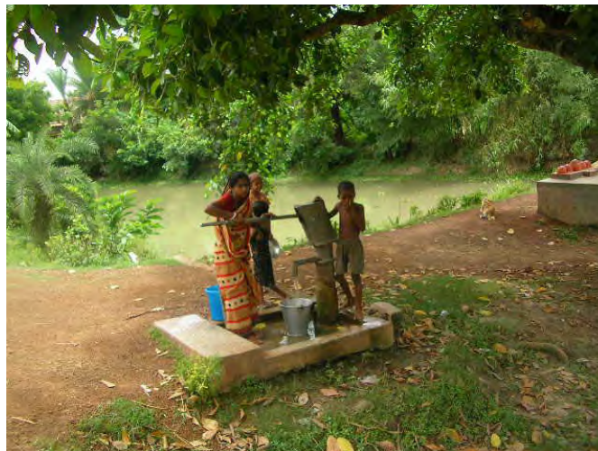
Figure 5.2.7 Hand-pump Well in the Kukurahati Area (photo taken on 1 July 2006)
