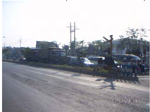
TANGGULANGIN (RAILWAY CROSSING)
