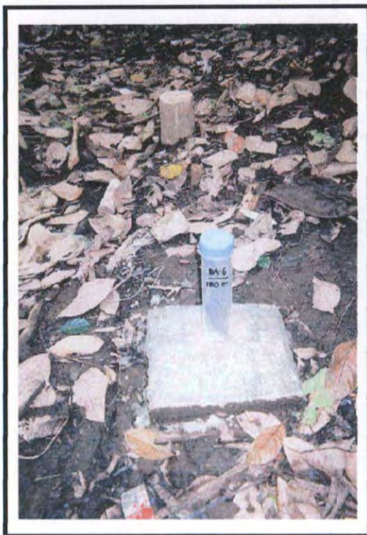
Open Stand Pipe Piezometer for DA-6
