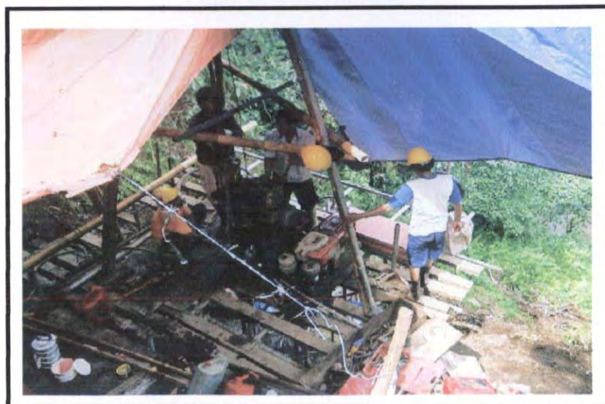
Drilling Activities at DA-10 Right Bank
