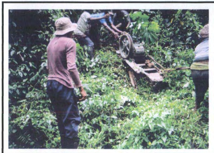
Moving Drilling Pump for DA-7 Drilling Preparation
