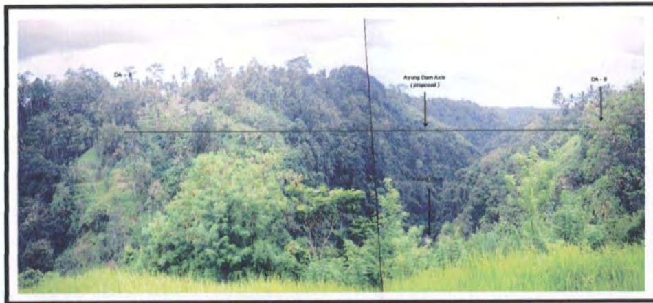
Location of Ayung Dam Site, Taken from the Right Bank
