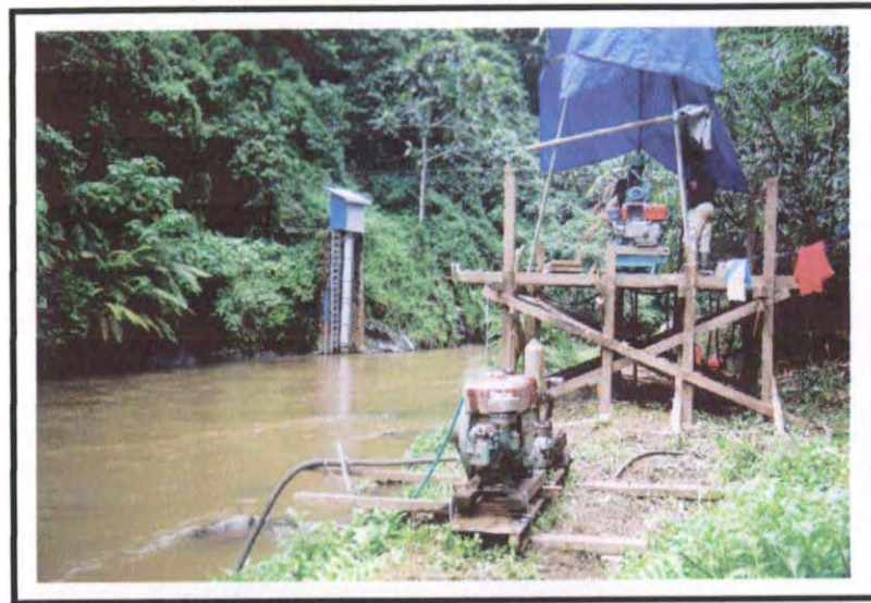
Drilling Activities at DA-7a
