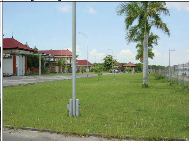
Estuary Water Treatment Plant
