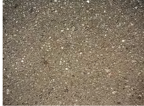
Pavement constructed 10 years ago with normal traffic
