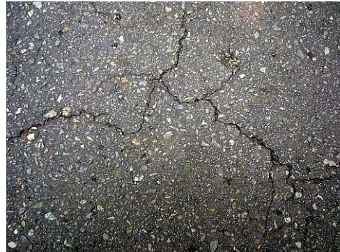
Pavement constructed 15 years ago with normal traffic
