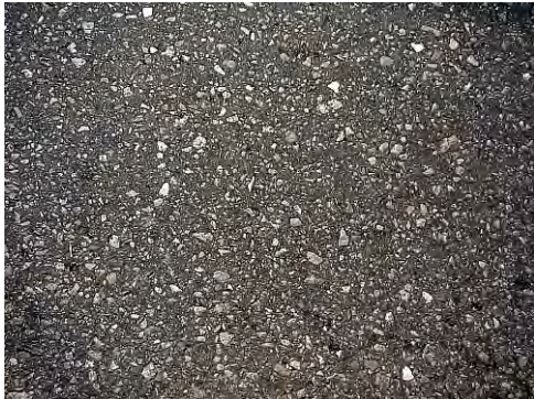
Pavement constructed 10 years ago with normal traffic
