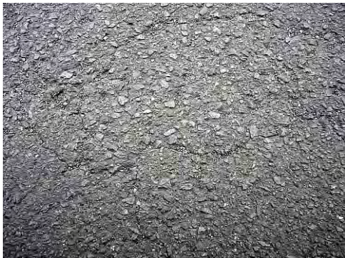
Pavement constructed 20 years ago with normal traffic
