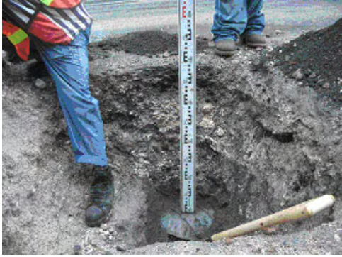
0.7 m deep steel pipe surrounded by 5 cm thick gravel
