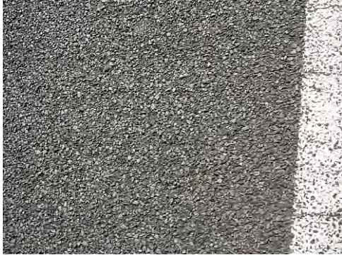
Storm-water penetration pavement constructed 4-5 years ago with heavy traffic
