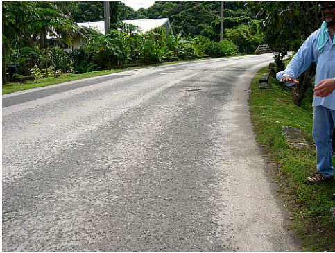
Section B STA. 2+400 Approach at Minato Bridge
