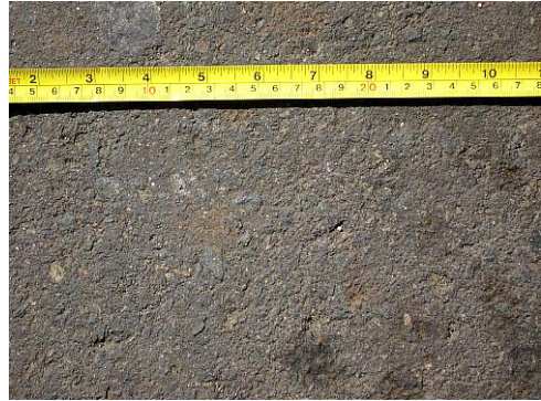
No damage at the area with roof
