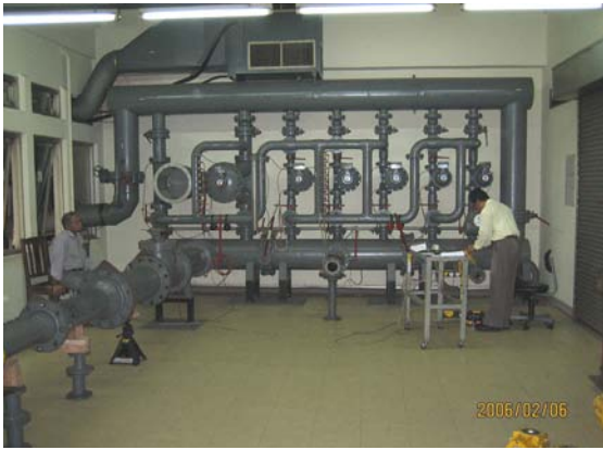
Photo 5.7.2.1 Gas meter calibration stand
