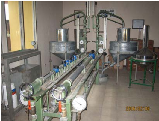
Photo 5.7.2.3 Water meter calibration stand
