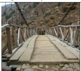
The existing suspension bridge was damaged by the earthquake in addition to damage from past floods and is now accessible only to foot traffic. Now vehicles must ford the river and this is not possible when it rains.
