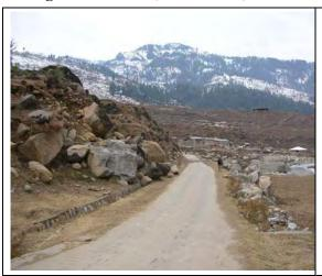
The road was located in the flat lands. Existing road width was around 5 m and that was suitable for two-way traffic. The road surface was double bituminous surface dressing. Damage to the road surface was progressing; however it was not in a serious condition. The traffic volume seemed large. There were a lot of hazardous areas due to land slides and fallen rocks.
