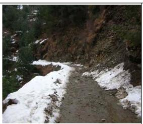
The road was located in the mountainous areas and had steep grades in places. The road width was 3-4 m equivalent to one traffic lane. In the hazardous areas due to slope failures, the road width was limited to about 2.5 m. That was insufficient for sedan cars. The road surface was soil and it was damaged. Traffic volume was quite small.
