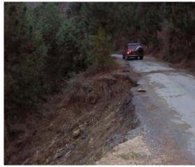
A lot of slope failures were observed at the upper and lower sides of the road
