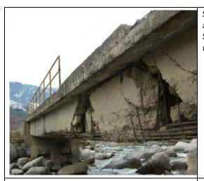
Superstructures are damaged and some parts of the reinforced concrete are exposed due to water pressure and floating debris when flooded. Sufficient clearance, especially consideration of the water level of floods, may be necessary before reconstruction.
