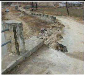
As it is supposed that the bridge and access roads are submerged during flooding, the access roads shall be reconstructed as Causeways.
