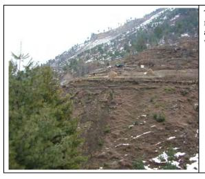
There were a lot of hazardous areas due to land slides and slope failures. In the rainy season, the road was frequently closed during and after the rainfall. The frequent closing caused a hindrance to the vehicular traffic.
