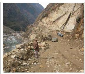
The road was located in the mountainous areas. The road width was 3-4 m equivalent to one traffic lane. In the hazardous areas of slope failures, the road width was limited to about 2.5 m that was insufficient for one traffic lane. The road surface was soil and damaged. Traffic volume seemed large. There were a lot of hazardous areas due to land sliding and slope failures. Great caution was required due to falling weathered stones.
