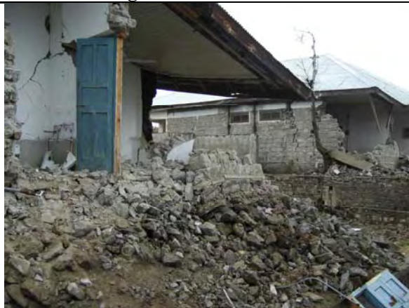
Greatly damaged OPD and Doctor's House
