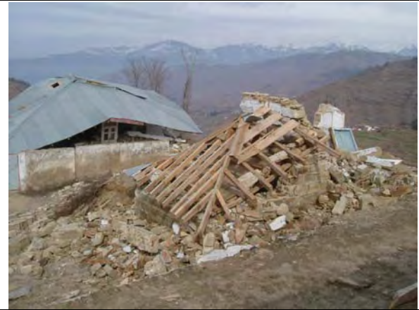
Collapsed staff house
