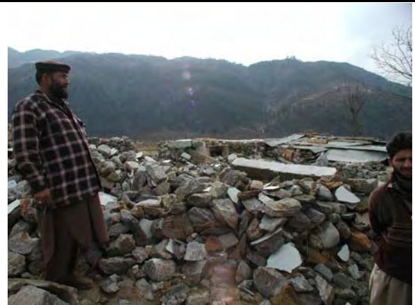
Collapsed staff house
