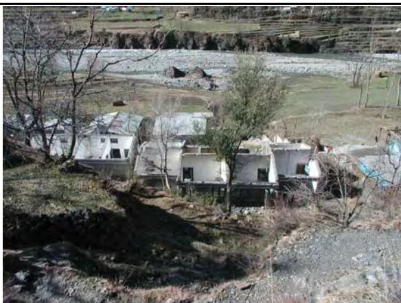
Panoramic view of hospital (All the roofs collapsed )
