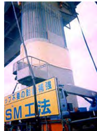
Figure 10-40 RC Jacketing Method
