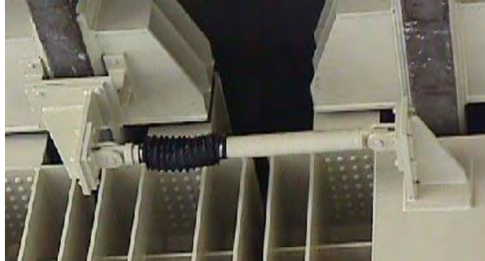
Figure 10-37 Example of Displacement Controlling by Damper
