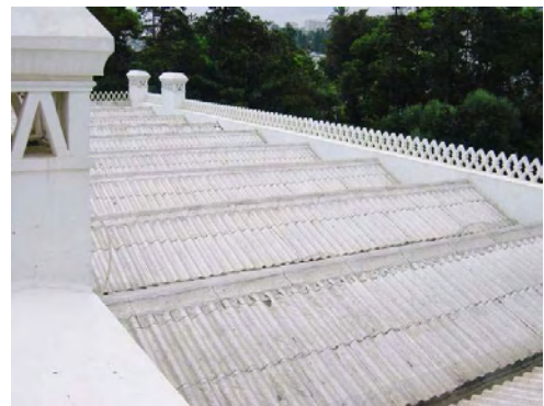
Photo 9-6 New Palace: Asbestos Roof for Main Hall
