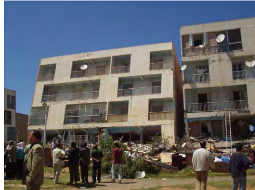
d) Destruction by Column Collapse
