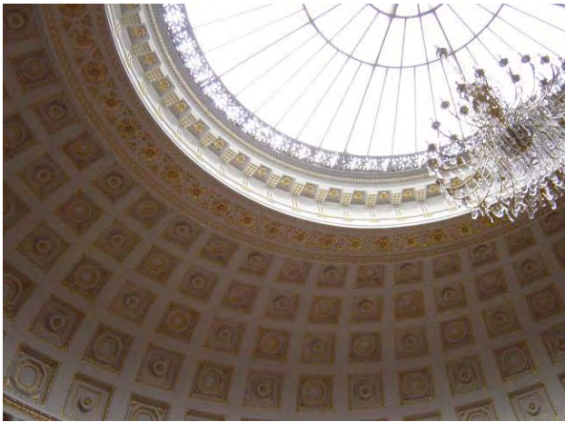
Photo 9-9 Top Light and Ceiling at Assembly Hall
