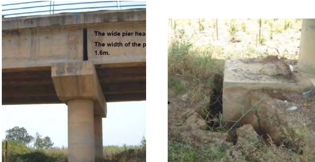
Figure 6-25 Displacement of a Girder and Lateral Movement of a Pier of SEBAO Bridge
