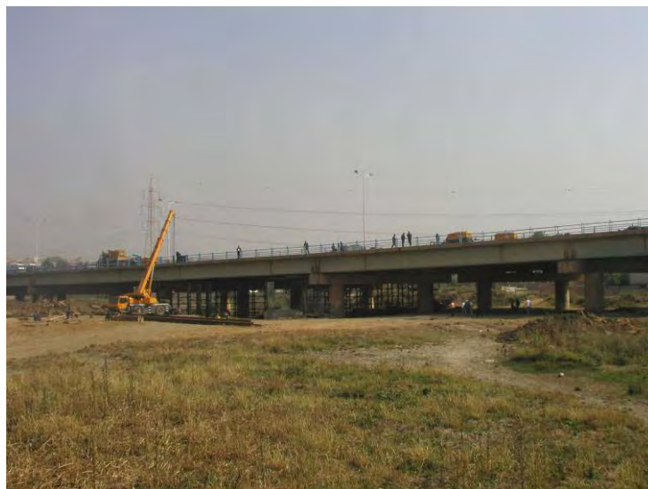
Figure 6-26 View of EL HARRACH Bridge
