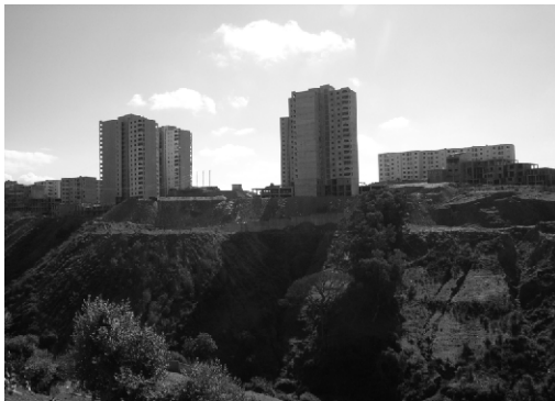
Photo 5-13 Unstable Soils along the River
