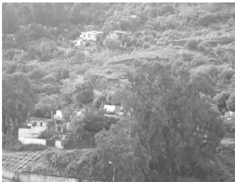
Photo 5-15 Slope along the Highway
