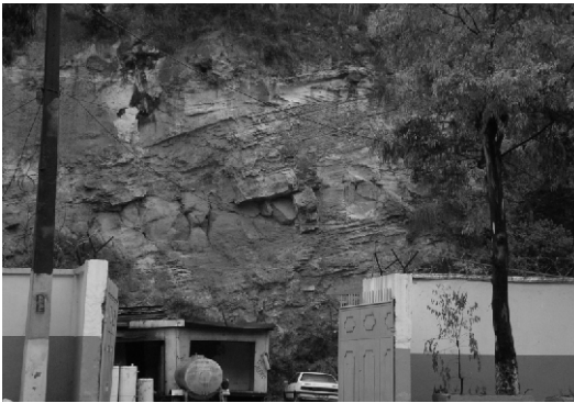
Photo 5-3 Slope Including Rock in the Wall
