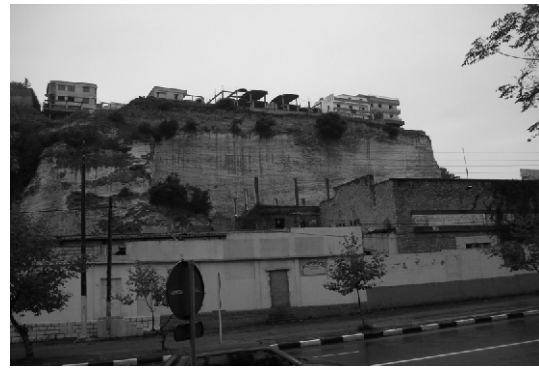
Photo 5-2 Houses at the Edge of Cutting
