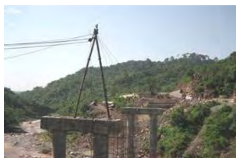
Photo: PC Beam Erection Method Common in Pakistan
