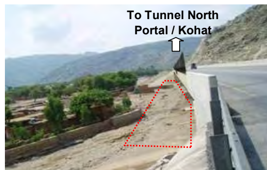
A Piece of Private Land located at No.6AR Bridge Construction Site (River Bed) at Sta.21+260
