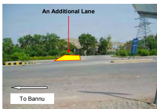
ROW for An Additional Lane Provision for Kohat Toi Intersection
