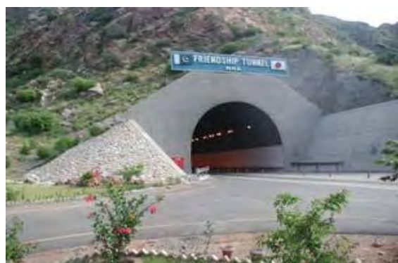
Kohat Tunnel South Portal
