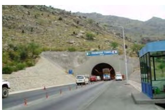
Kohat Tunnel North Portal
