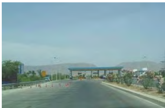
Main Toll Plaza at Sta.10+600
