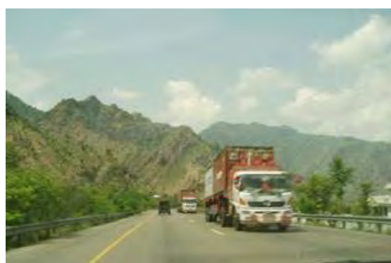
Access Road in Tunnel North Section
