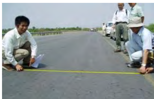
Minor Rutting (Depth 5-10mm)
