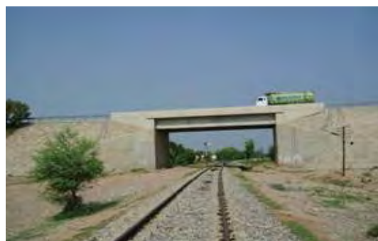
Bridge No.3A (L=20 m)
