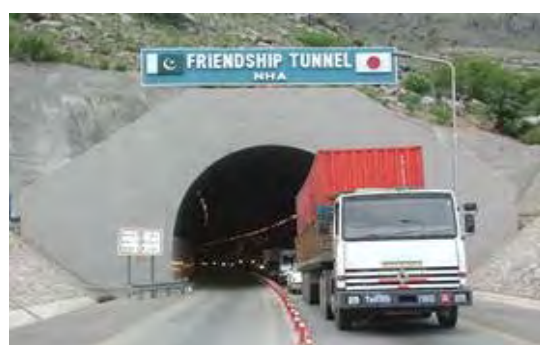
Slow Movement of Traffic at North Portal
