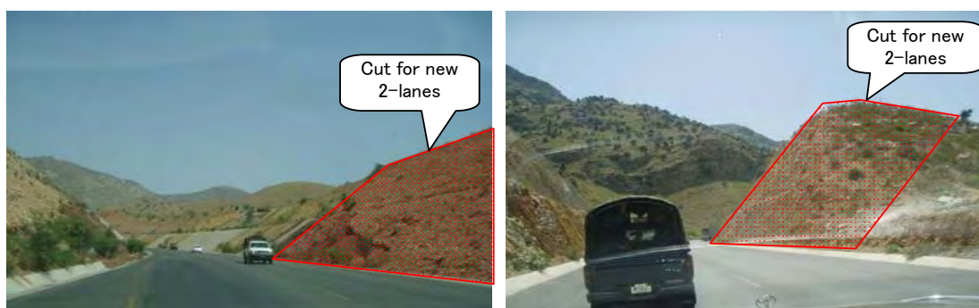
High Cut in South Section At Sta.18+100 -Sta.18+700
