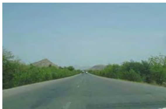
Access Road in Tunnel South Section
