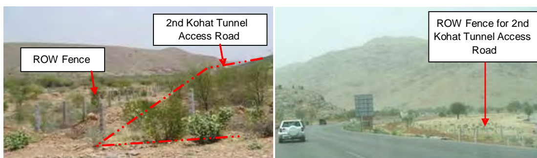
Existing ROW Fence for the 2 nd Kohat Tunnel Access Road
