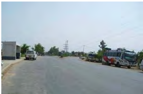
Kohat Toi Intersection (Start Point)
