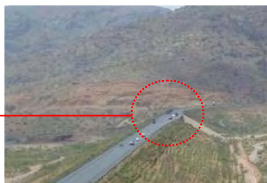
Bridge No.4 already constructed as a 4-lane bridge
