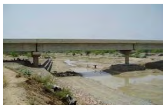
Scouring Repair Works by Gabion for Bridge No.1
