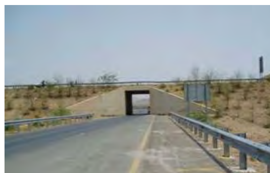
Kohat Link Road Off-Ramp, Narrow Box-culvert for Underpass
