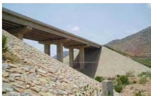
Bridge No.4 (L=120 m, Pier Height=30 m)
