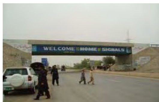
Bridge No.3B (L=30 m)
