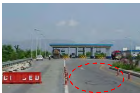
Weigh Bridge at Main Toll Plaza
