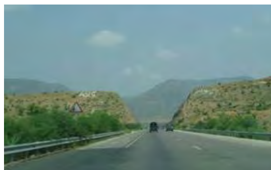
Repair of Damaged Shoulders
